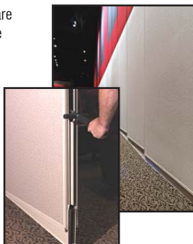
Although the panels range in height to 32', they can be easily moved into position when needed or stored in a nearby pocket when the entire facility is used. The panel finish matches the permanent walls.
